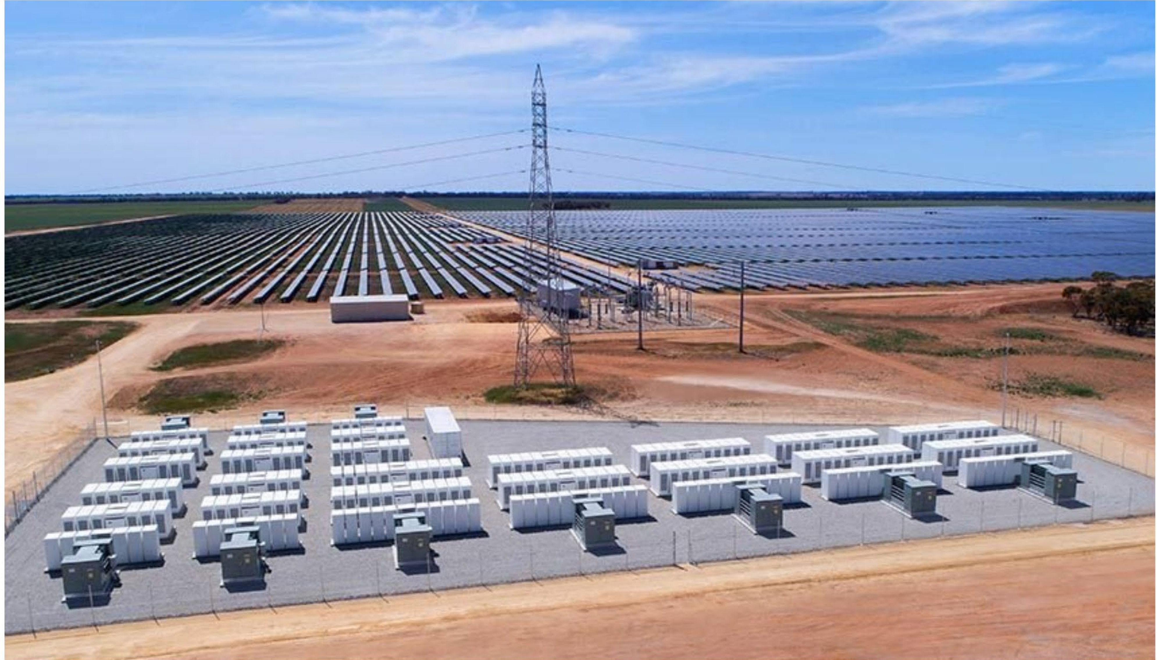
Gannawarra Energy Storage System
