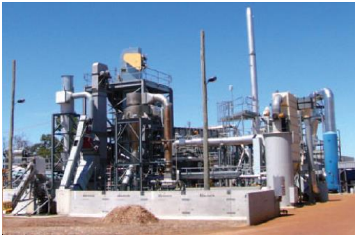
Gas-fired power plant
