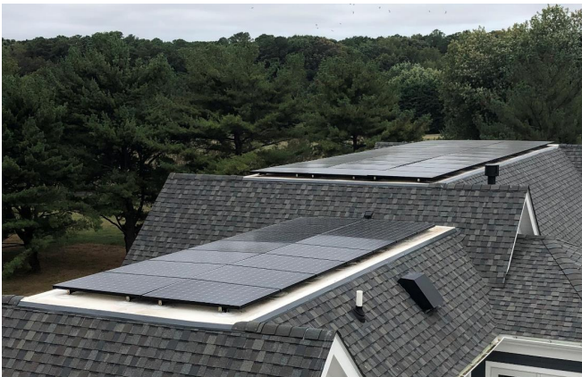
Figure 3 Solar PV array atop the house
