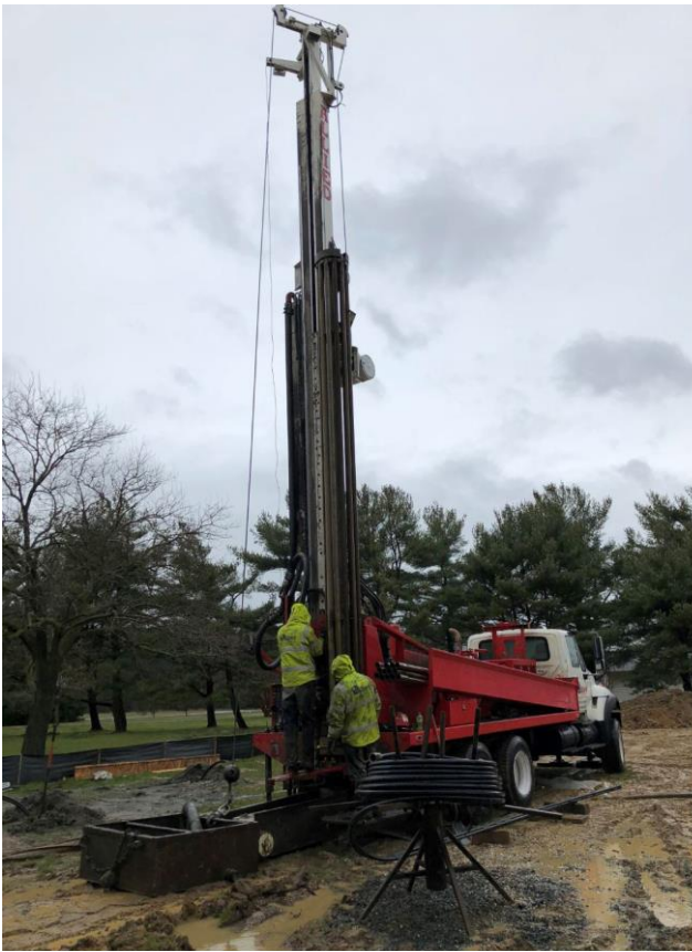
Figure 2 Geothermal drilling underway on property
